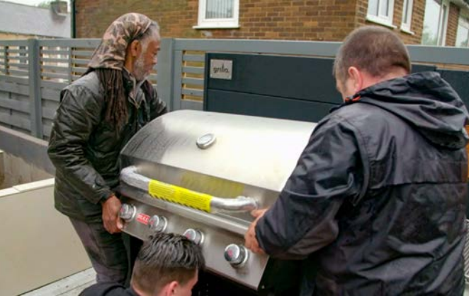
Danny Clarke gives the Grillo install team a helping hand. If you're ever looking for a new job, Danny...
